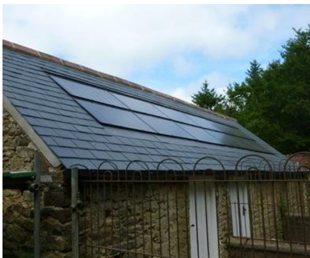
Figure 2: Example of in-roof (integrated) PV panels
